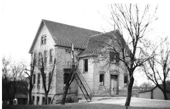
St. Theresa School (2 nd building)
